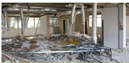
TRADITIONAL CONSTRUCTION SITE
