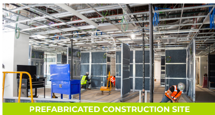
PREFABRICATED CONSTRUCTION SITE
